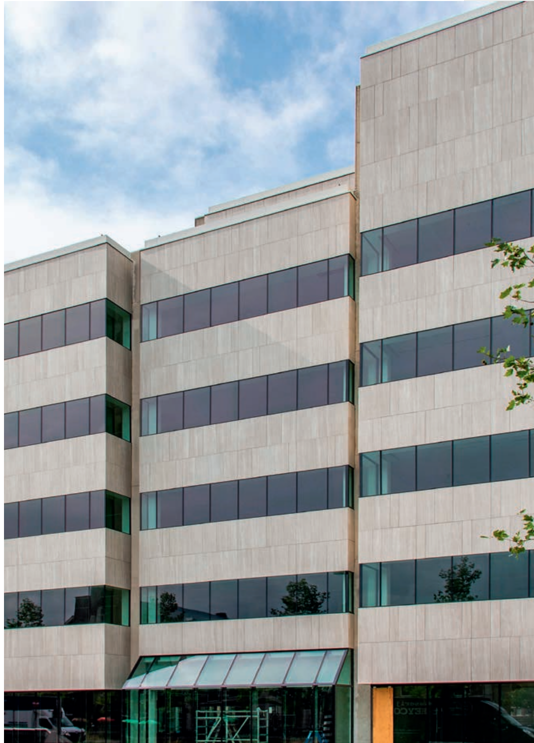
ABN AMRO BUILDING, Utrecht, (Netherlands)
